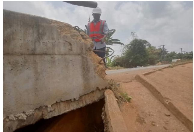
Figure 5: Visual inspection of the Orogodo Composite Bridge
