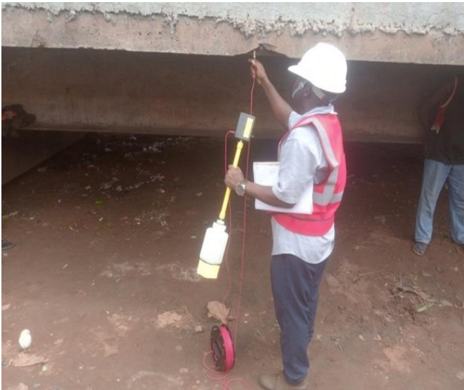
Figure 13: HCP Test Connection on the Orogodo Bridge Deck
