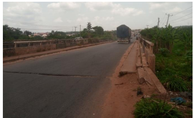
Figure 2: The Existing Orogodo Composite Bridge
