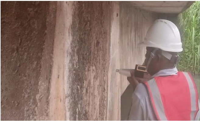
Figure 8: Digital Rebound Hammer test on Orogodo Composite Bridge
